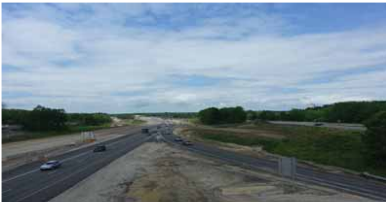
Contract M - Southbound Construction at Exit 3
