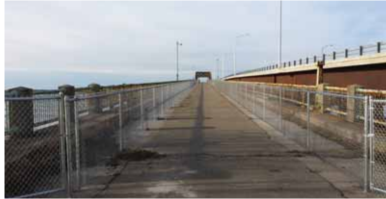
Reduced Width General Sullivan Bridge
