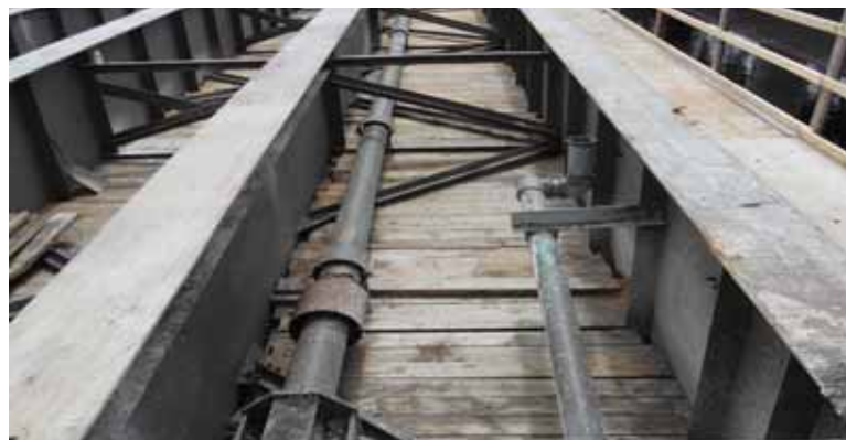
Contract O - Existing Little Bay Bridge Structural Steel and Utility Pipes
