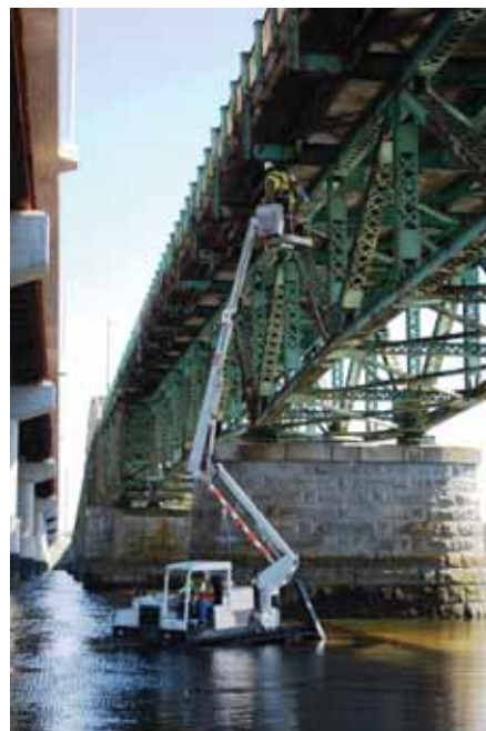
Bridge Inspection Activities at Low Tide
