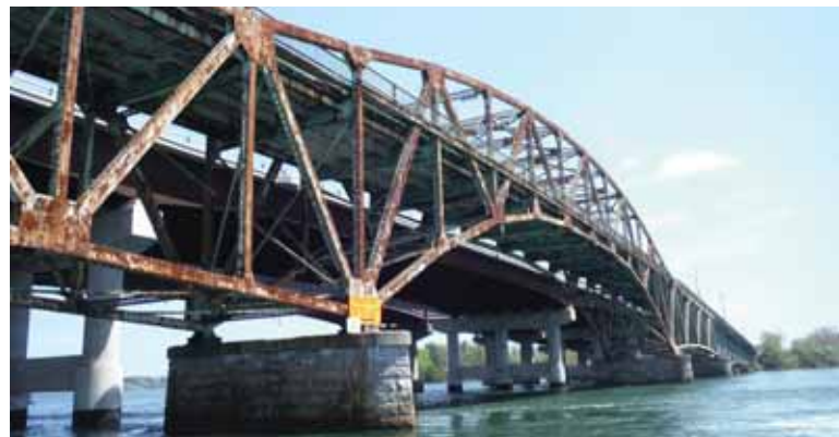
Iconic Metal Truss of General Sullivan Bridge
