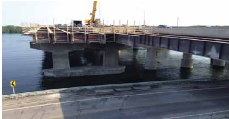
Contract O - Existing Little Bay Bridge over Wentworth Terrace
